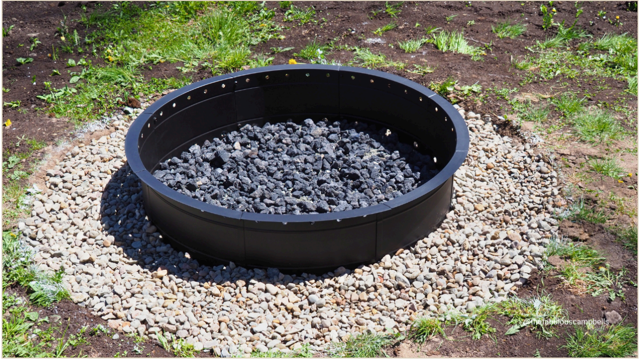
The final result—clean lines, solid drainage, and ready for wood and a match.
