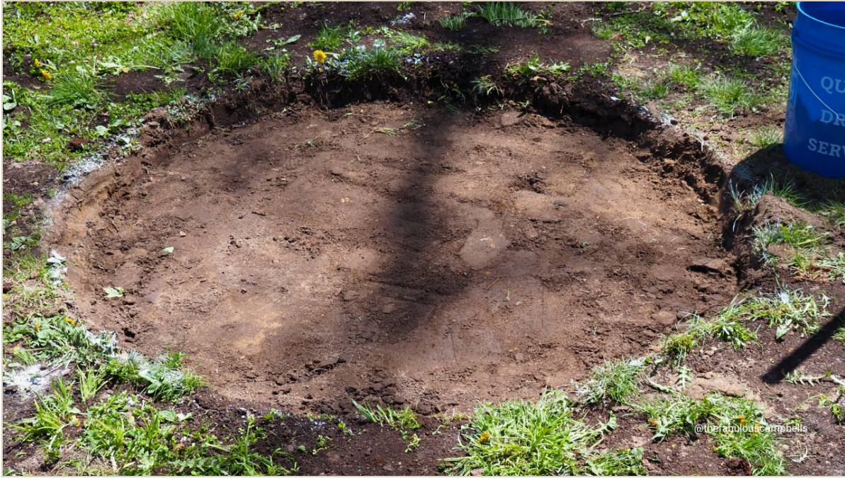
Clearing away the heavy sod down to a flat, 3-inch recessed basin.
